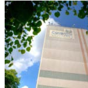
Coventry University George Eliot Building (Coventry, UK)
