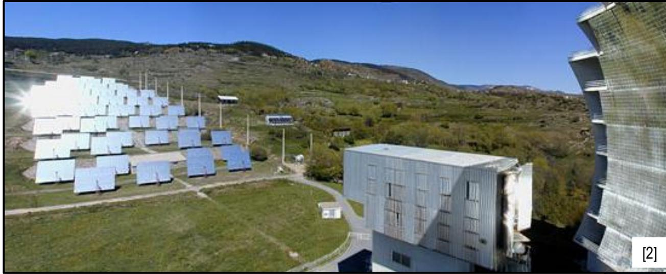
CNRS-PROMES's 1 MW Solar Furnace in Odeillo, France, is a globally unique Research Infrastructure (RI) used to advance the state-of-the-art in materials and process research requiring extreme heat fluxes and temperatures.
